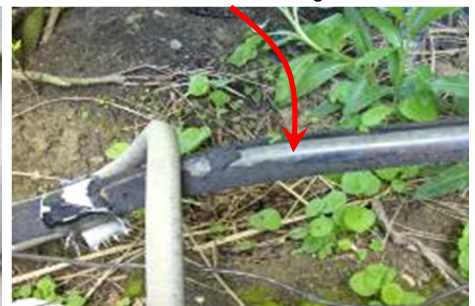
Bad insulation on cooling line
