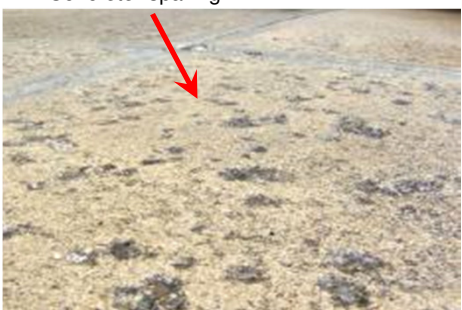
Concrete "spalling".
