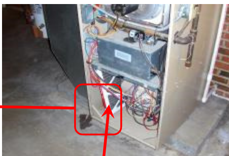
Furnace Filter Location
